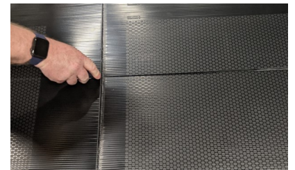
3. Cut along flute with the aid of a straight or hooked blade
