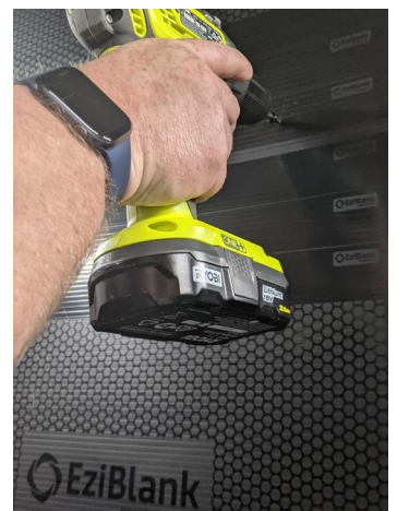
6. Secure new section with self tapping screw
